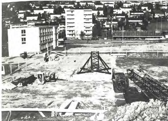
November 1978, Baustelleninstallation / installation de chantier
