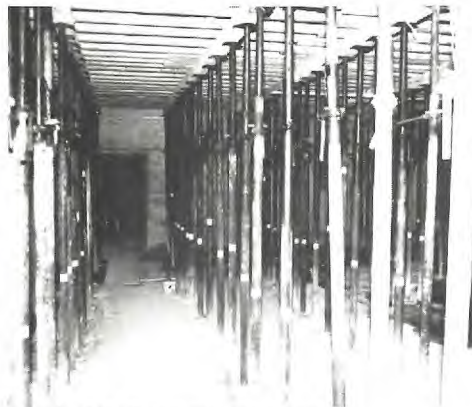
August 1979, Schiesskeller / sous-sol aile "Sport"
